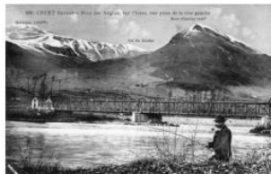
Figure 3. Railway bridge over the River Isère near Crucet: the continuous wrought iron truss (Goutagny Postcard 1889).
