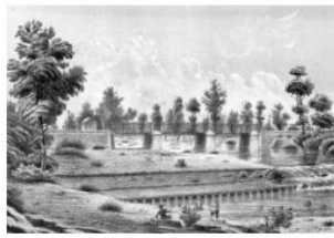
Figure 2. Railway bridge near Novara: the piers built in 1855 by the same company of Rochester Bridge (Fassò 1880).
